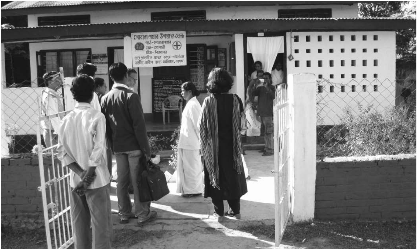
This Sub-centre in Assam, was having a poor delivery case load, may serve as Type A Sub-Centre.
